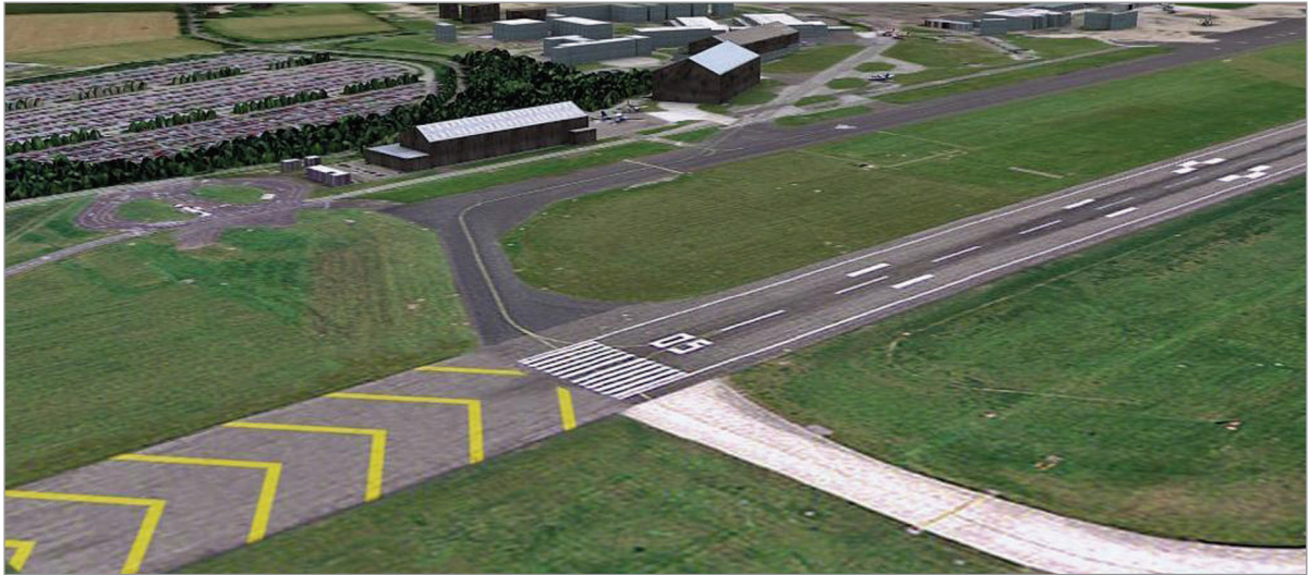
Figure 2.2 Stopways are able to support the aeroplane during a rejected take-off and are marked by large yellow chevrons
