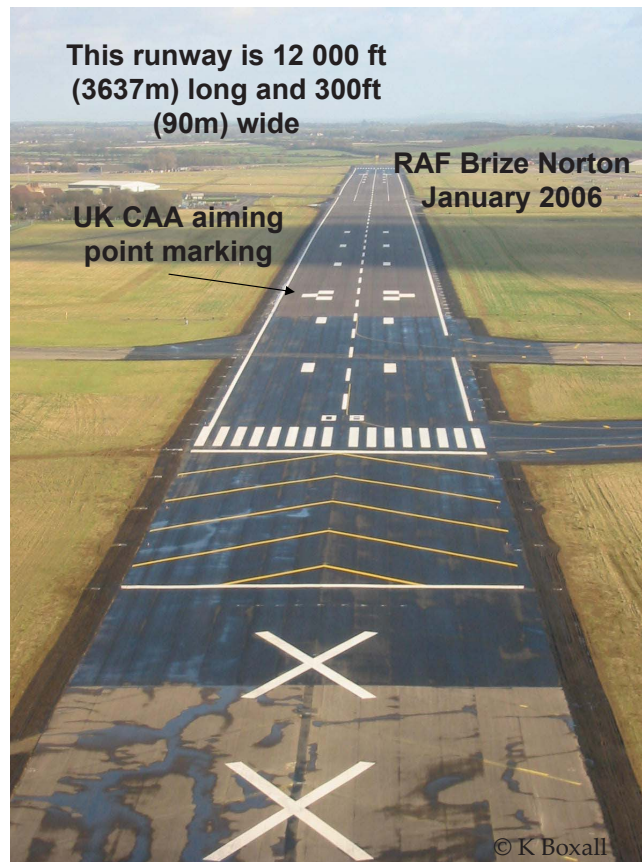
Figure 20.1: Runway markings at RAF Brize Norton.
