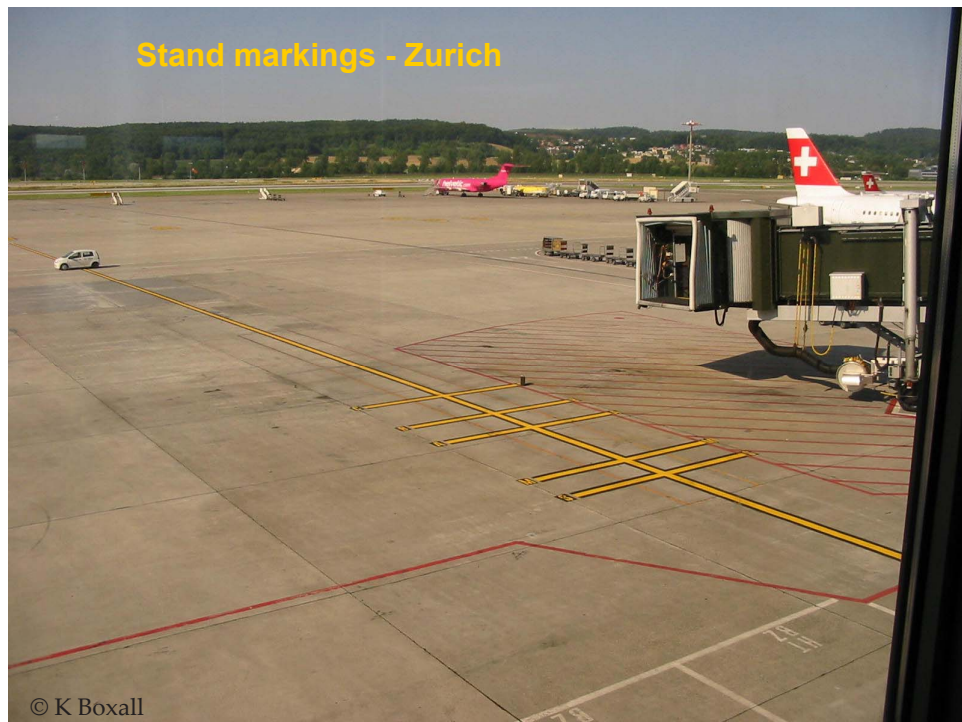
Figure 20.11: Aircraft stand markings.
