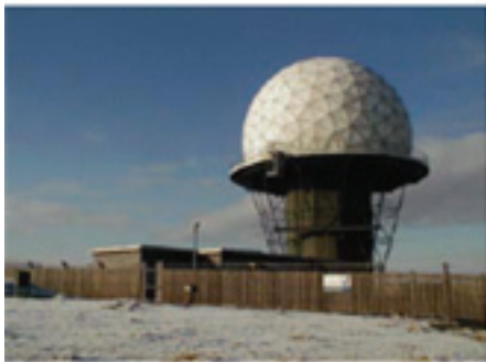
Figure 17.1: ATC radar head at Cleve Hill, Shropshire.
