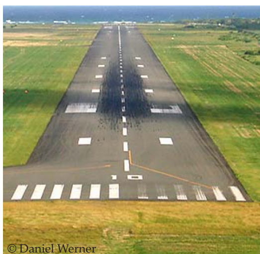
Figure 20.5a: Pattern "A", basic plain markings.
