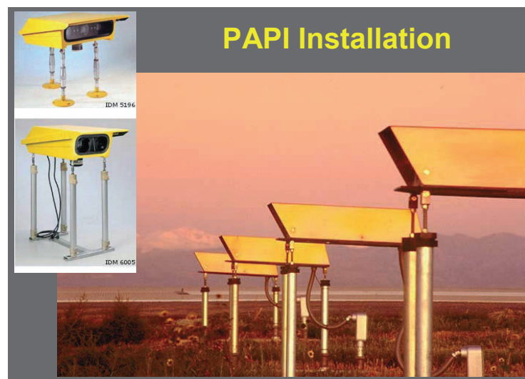
Figure 21.7: Precision approach path indicators (PAPI).
